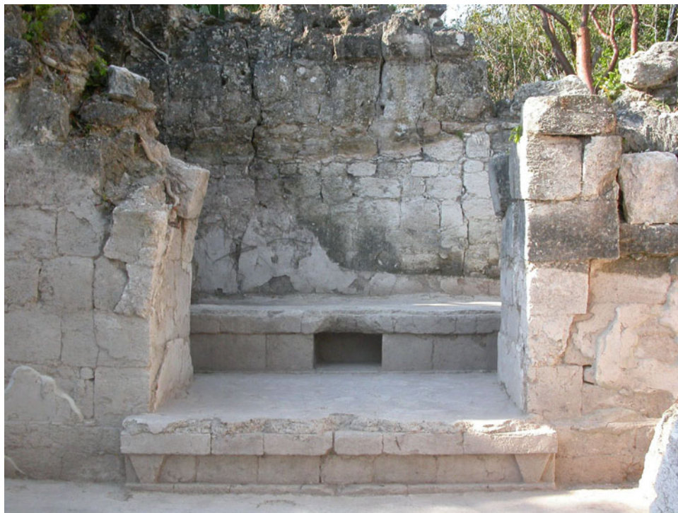
Figure 11. Río Bec, Group D, Structure 7N1. The step to the inner room is decorated with legs imitating a wooden bench. On its raised floor, the inner room has a masonry bench with a niche [before consolidation]. Note curtain holders holes plugged on the sides of the doorway. Photo courtesy of the Proje Río Bec.
